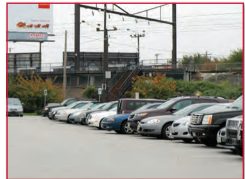
West Baltimore MARC Station
